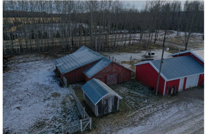
BARN 25x50 plus side lean to. Wood frame and exterior Power 2 Hydrants 3 Livestock waterers
