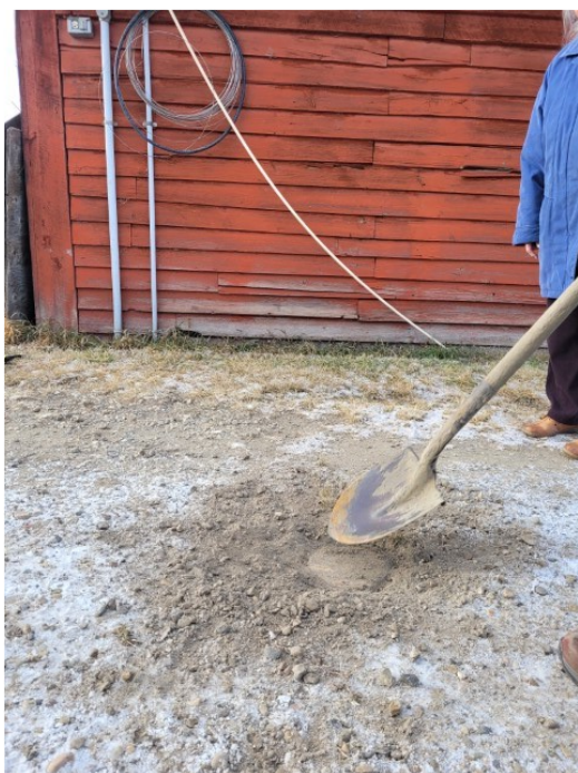
Access to underground tank for used oil - 4x4x8 constructed of 3/8" steel plate
