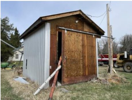
Metal clad shed with slide door and concrete floor.
