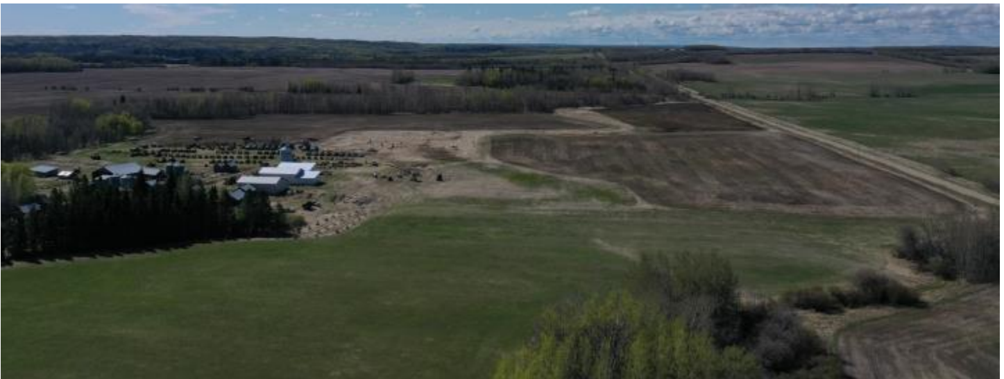
Northwest corner looking south
