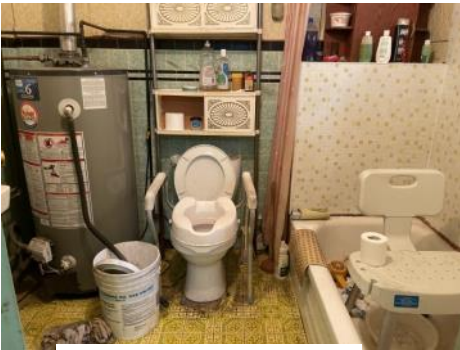
Bathroom in addition
