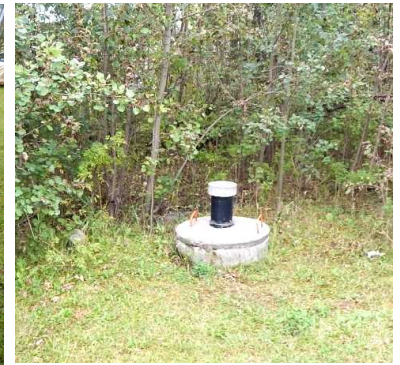
Sewer holding tanks for home
