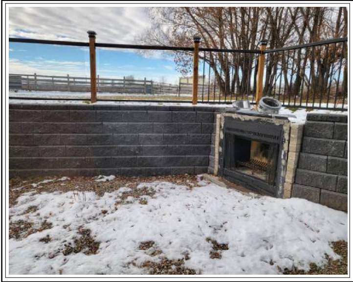
Patio with wood burning fireplace
