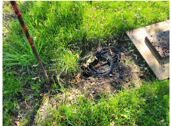
Heat Tape for thawing culvert in spring.
