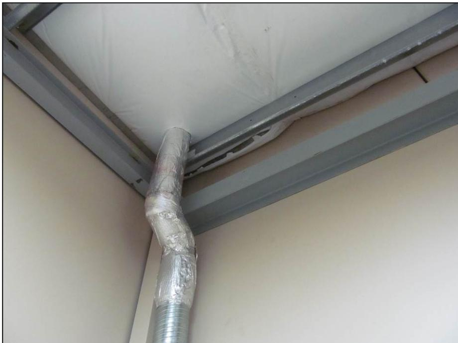
Photo #8: Potential location for mold growth from former leaking roof in northeast corner of bay 4, building 569.
