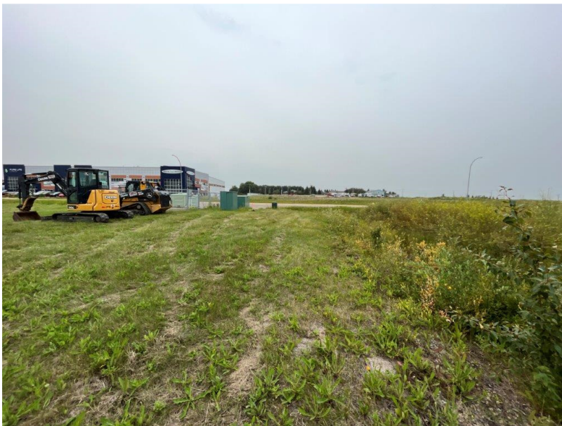
Photograph 1: Looking west to the Liberty Sanitary Lift Station in the northwest corner of the Property.
