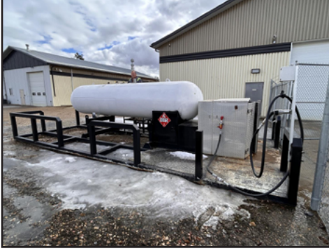
Propane Filling Station with Tank On Skid
