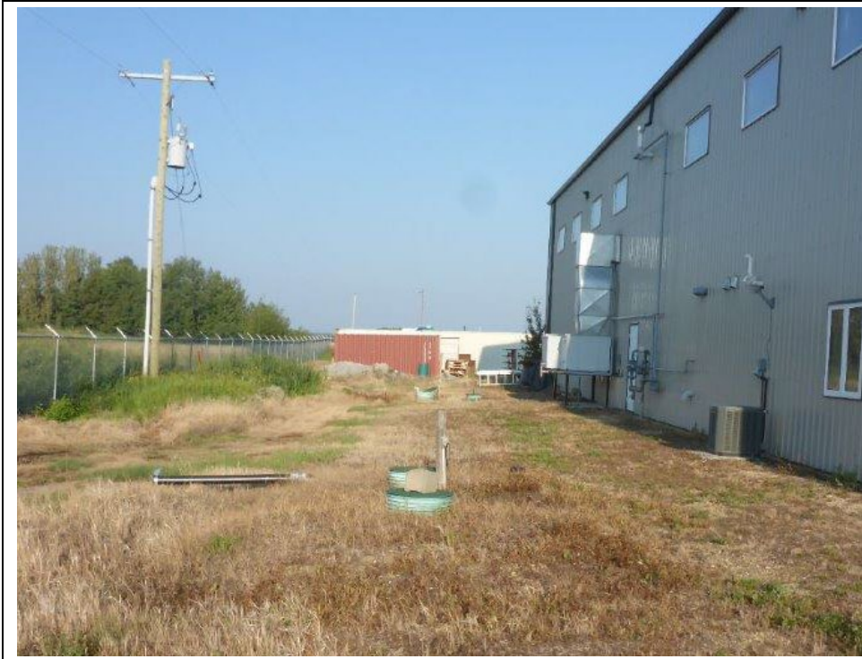
Photograph 9: Southern portion of the Site showing infrastructure associated with a well (foreground) and septic tank (background). An approximately 15,000 L underground storage tank located in this area collects rainwater from the building roof for use in the wash bay.
