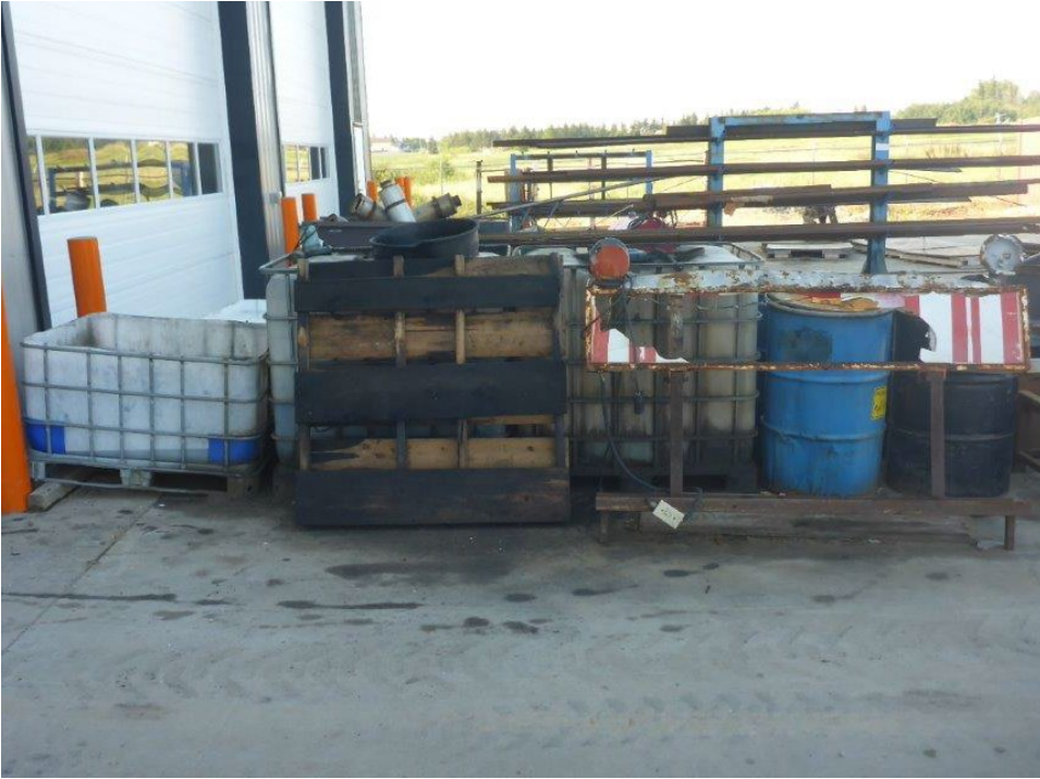
Photograph 15: Waste oil generated from vehicle maintenance is collected in two IBCs located on the concrete pad outside the west side of the building. Drums used for the collection of oily rags, spent oil filters and emptied oil containers were also present in this area. Staining was visible on the concrete pad in this area.
