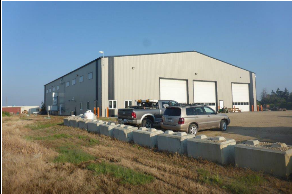
Photograph 1: The Site building as viewed from the southeast.
