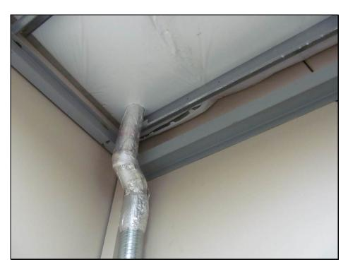
Photo #8: Potential location for mold growth from former leaking roof in northeast corner of bay 4, building 569.
