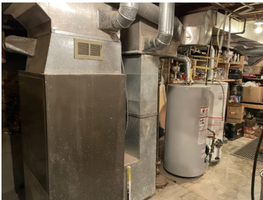
Forced air furnace provides heat to both the store area and the suite.
