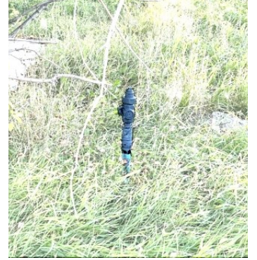
Gas Riser - located east of barn Cost $42 +/- per month Meter needs to be installed.
