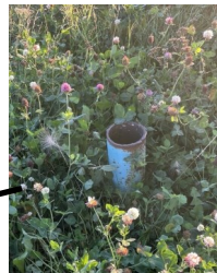
20' Steel pilings in ground east of barn - 16' diameter for mounting round grain bin.
