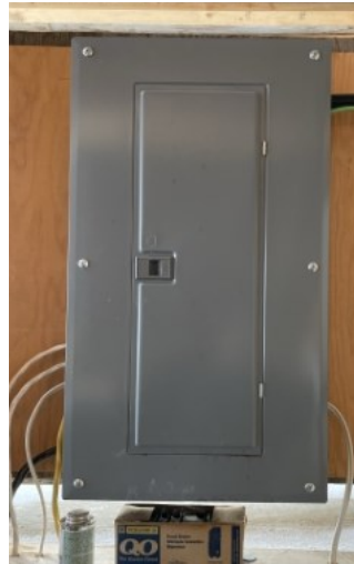
Electric panel is installed. Extra breakers included
