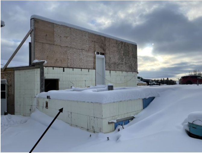
Footings and basement ICF wall for future garage and wine cellar / cold room.
