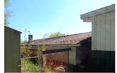
Shingles on north side of shop are in need of replacement.
