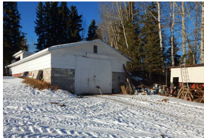
24x54 shop - constructed with cinder block pony wall & is wood framed from pony wall to ceiling. Large hinged doors with man door on the left large hinged door. Concrete floor, overhead heater (hot water heat from outside boiler) & has 220 wiring. Wood benches and wood bolt bin included. Peg boards excluded.
