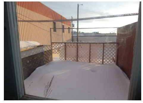
Deck off apartment. Air conditioning unit for restaurant located on deck
