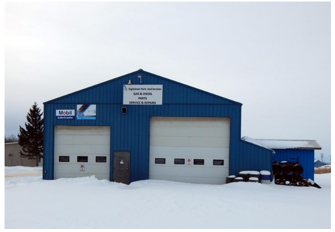
East end of building - showing doors into the shop area.
