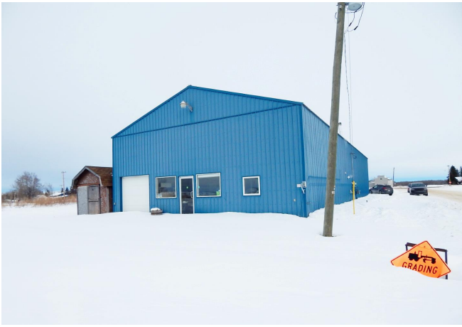
West end of building - showing doors into the front retail area.
