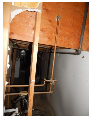
Former 3 piece bath in basement - the walls & shower were demolished to allow for install of the interior weeping tile system. Drain remains in place as well as the water pipes.
