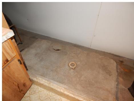
Former 3 piece bath in basement - the walls & shower were demolished to allow for install of the interior weeping tile system. Drain remains in place as well as the water pipes.
