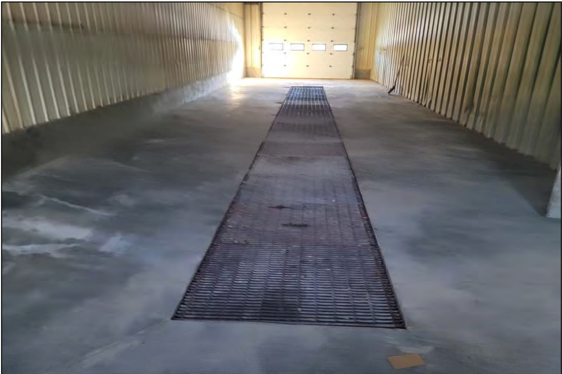
Photograph 8: Looking at the wash bay (Oct-25-23).
