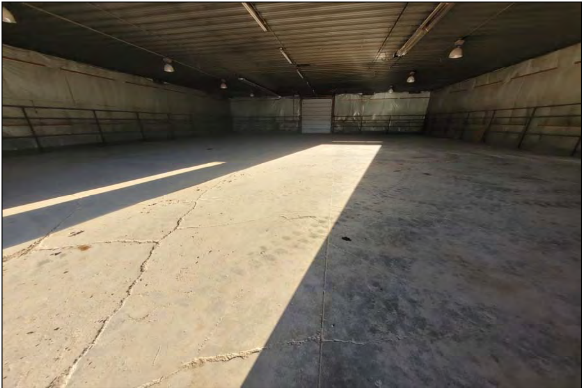
Photograph 12: Looking at an empty bay (Oct-25-23).
