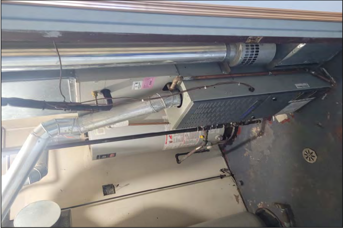
Photograph 7: Looking at utility room (Oct-25-23).
