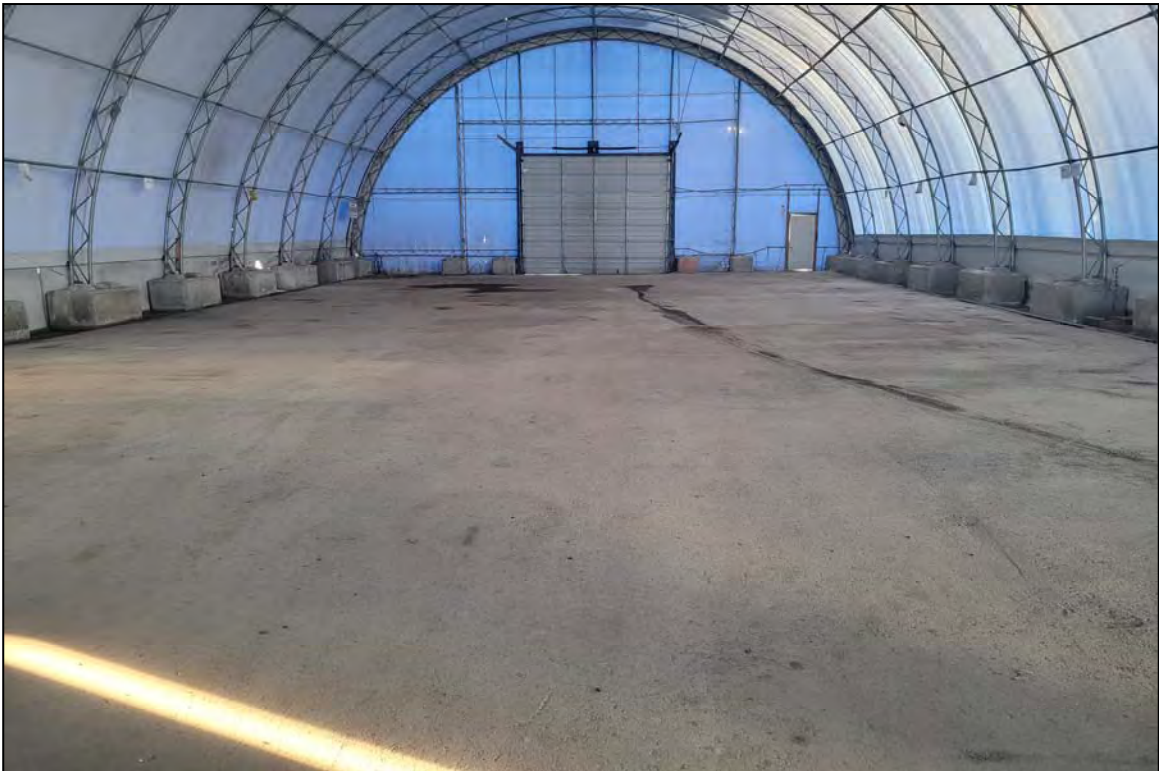
Photograph 10: Looking inside of canvas building (Oct-25-23).
