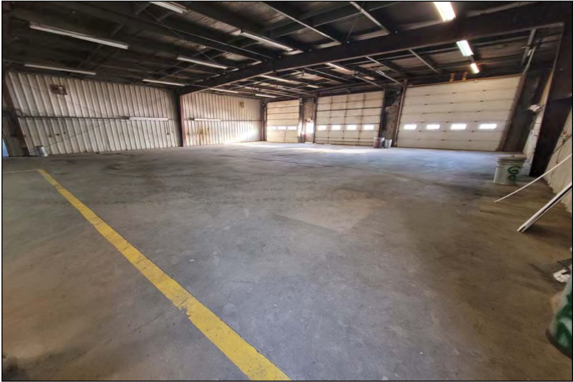
Photograph 5: Looking at the bay in the main building (Oct-25-23).
