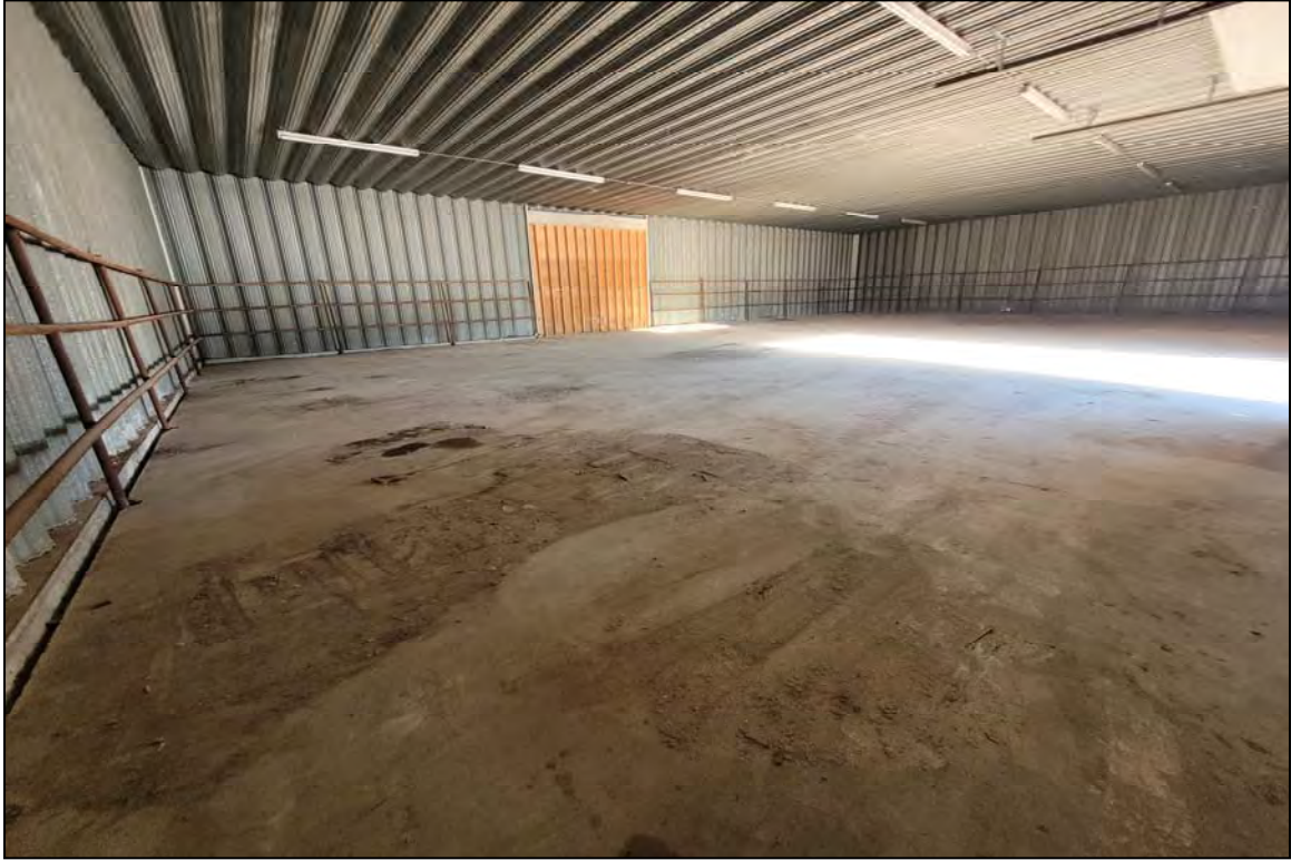
Photograph 11: Looking at an empty bay (Oct-25-23).
